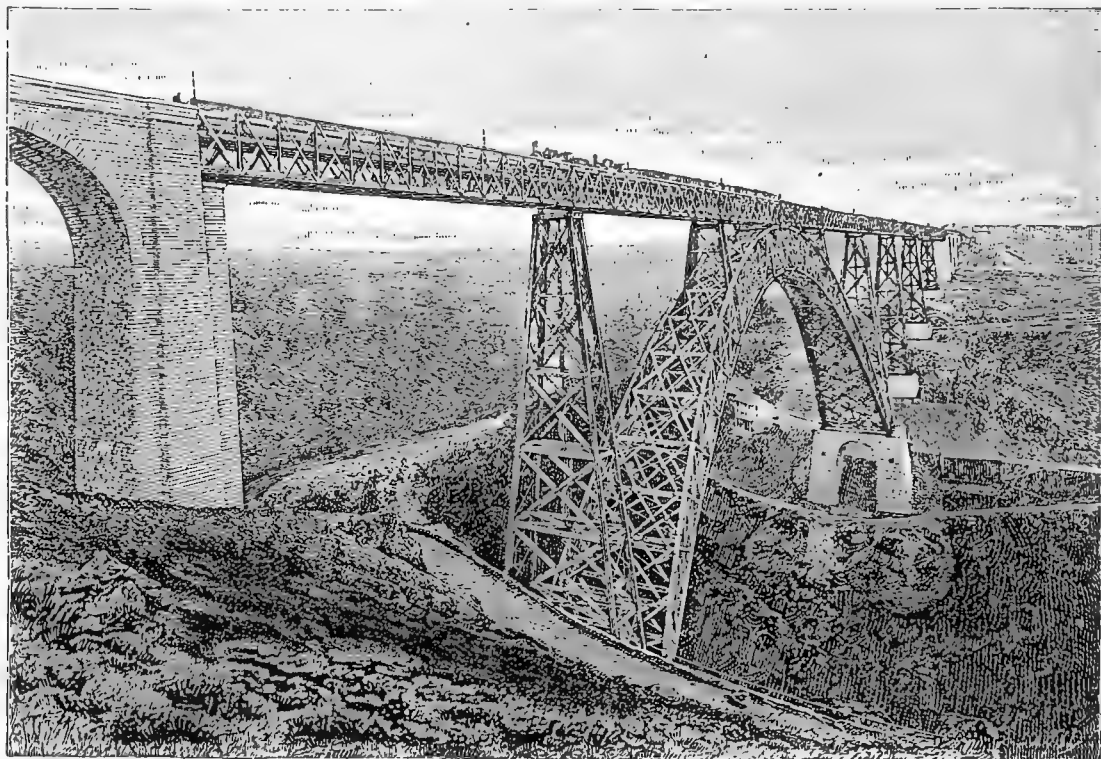
FIG. 4.—GENERAL VIEW OF THE VIADUCT OF GARABIT.
